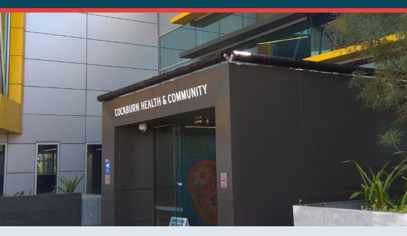
Roller Guard is the non-aggressive anti climb system of choice for use where children or vulnerable people are present. This non-aggressive Roller Spinner system is the Anti Climb Barrier that offers practical and effective perimeter security - without the risk of intruders impaling or seriously injuring themselves on other climb products, like spiked products, barbed wire and razor wire.
